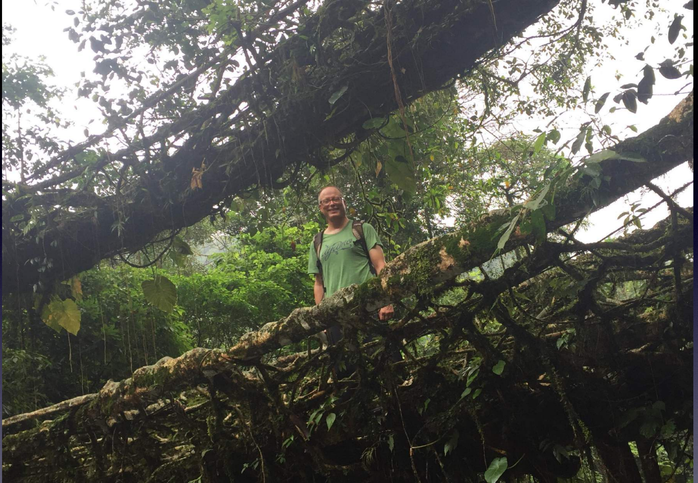
On the bridge from below
